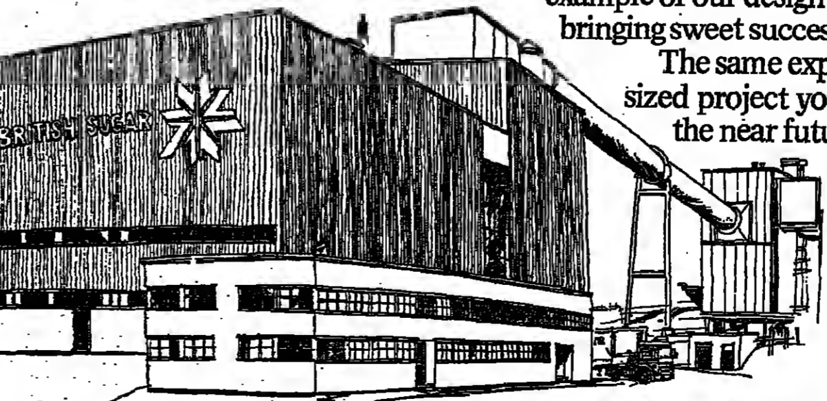
One of Europe's largest and most sophisticated sugar packaging and distribution complexes. Fully automated with the very latest management computer and micro-processor system.
